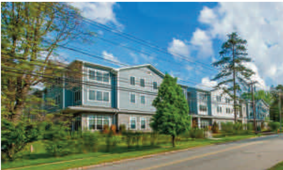
Sacred Heart Convent, 40 Ryerson Avenue, Caldwell. To learn more about environmentally-conscious and elder-friendly construction throughout, please visit www.caldwellop.org/SacredHeartConvent.php and download our brochure.
